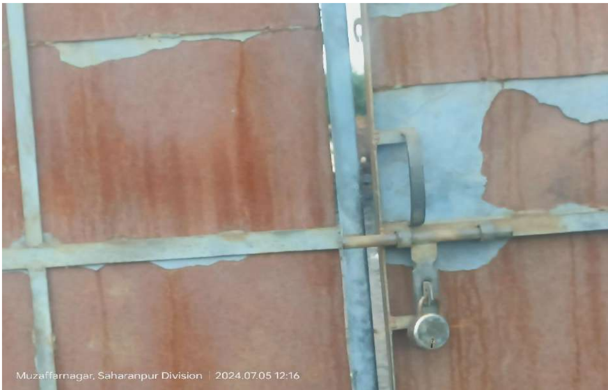
Figure 2 Lock at main entrance gate
