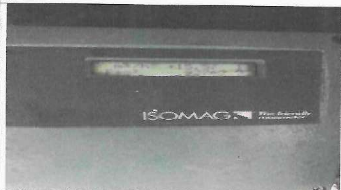
Photo 7: Flowmeter at recycling line after sedicell
