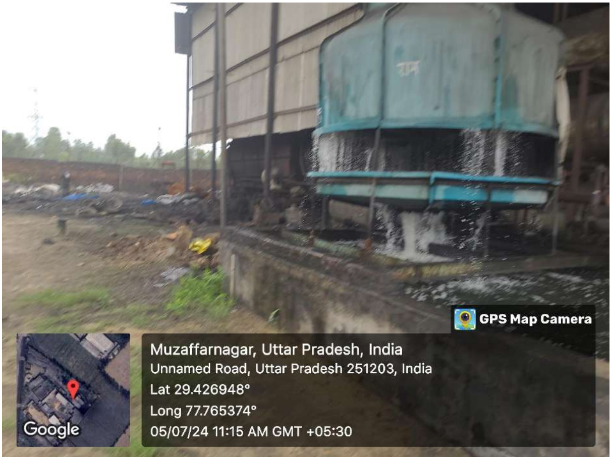
Figure 8 Cooling Tower
