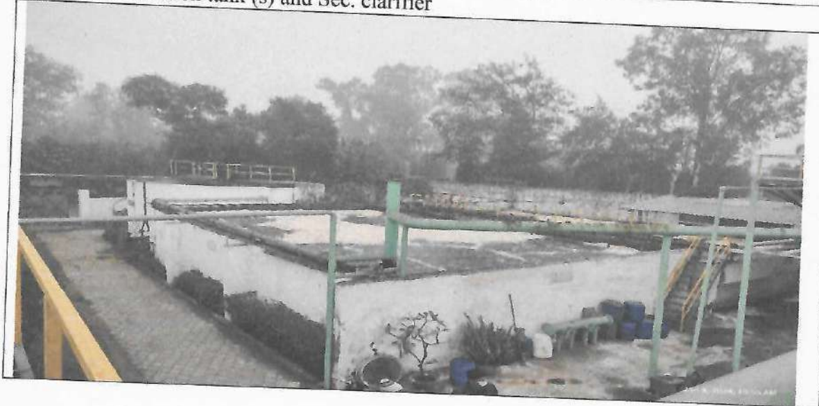
Photo 10: Aeration tank (s) and Sec. clarifier
