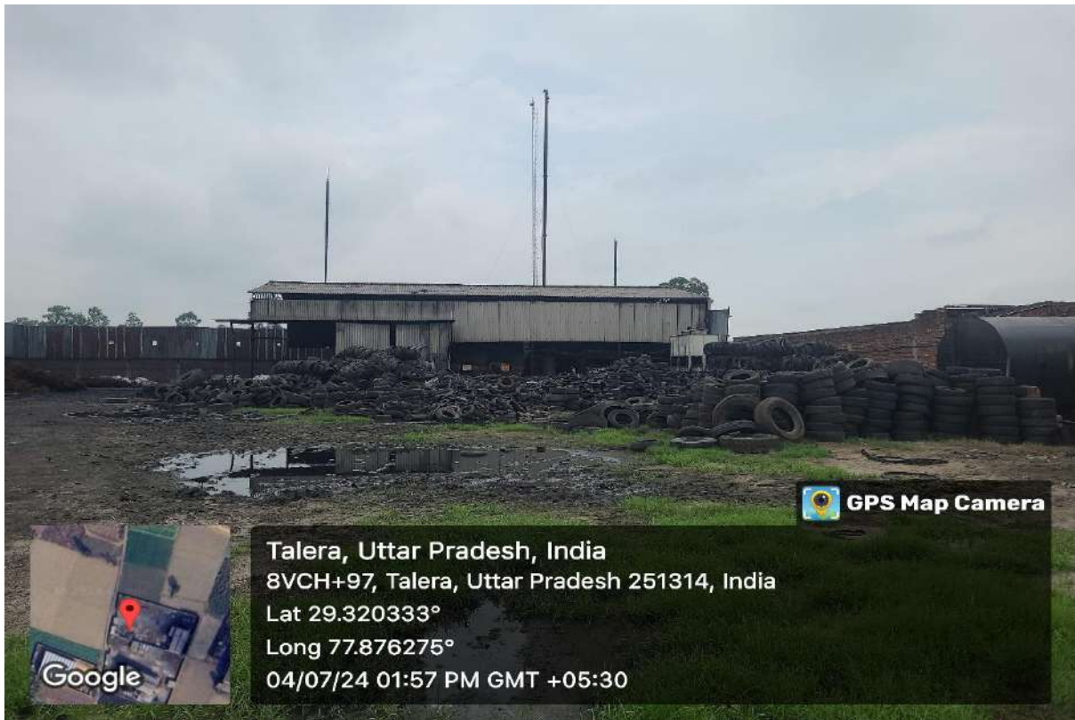
Figure 2 Unit premises and stored tyres inside premises
