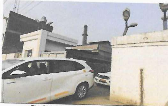
Fig.2: Manufacturing Process area
