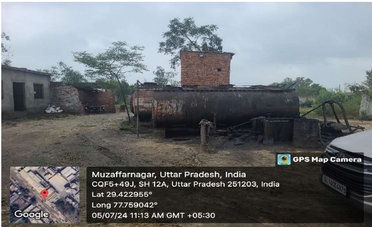
Figure 2 Unit Premises and Oil tanks
