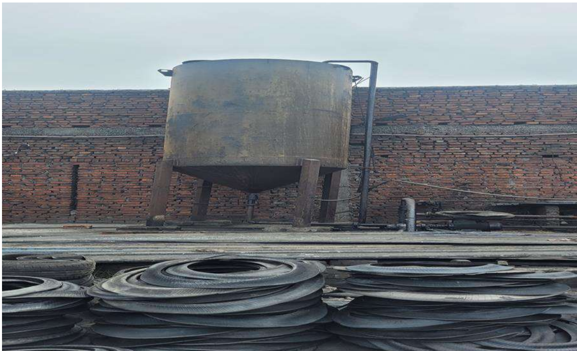
Figure 6 Pyro Oil storage and filter
