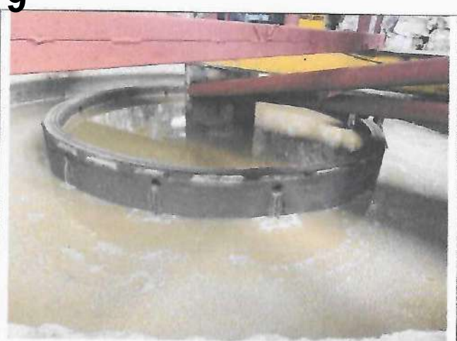
Photo 6: Overflow tank cum storage for recycling
