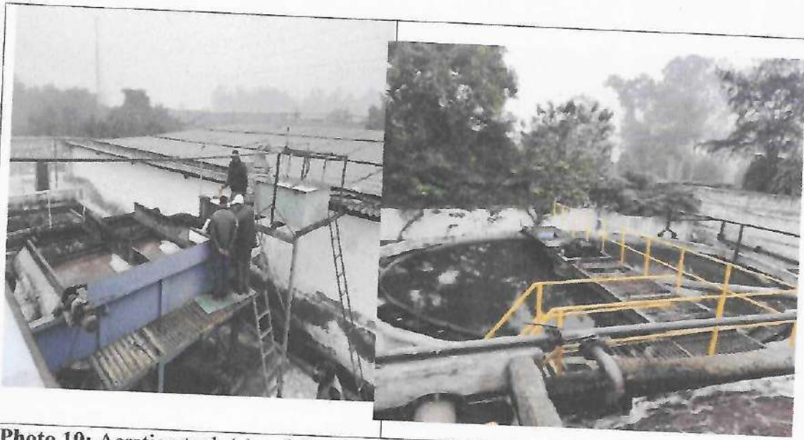
Photo 10: Aeration tank (s) and Sec. clarifier
