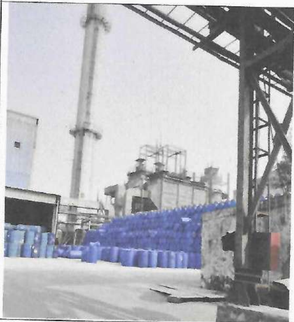
Fig.10: APC system and Stack attached to Boiler
