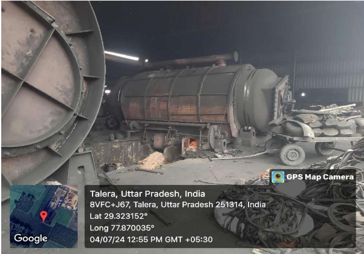
Figure 5 Pyro-reactor running at the time of inspection
