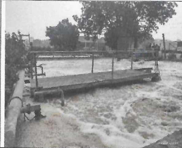
Fig.5: Aeration tank
