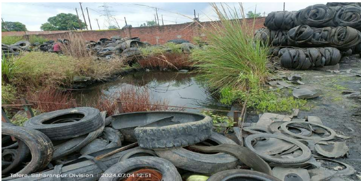
Figure 10 Ponding of wastewater inside unit premises.
