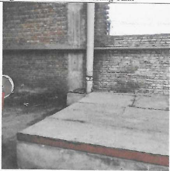
Fig.16: Rain Water Harvesting Tank
