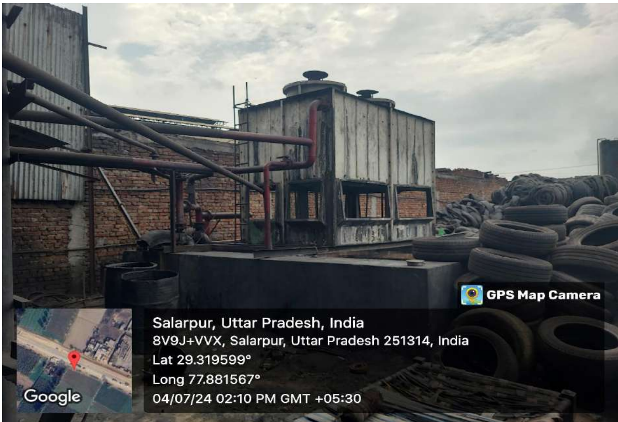
Figure 9 Cooling Tower
