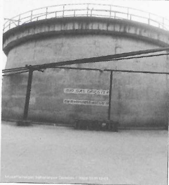
Fig.4: Bio-digester (Anaerobic Treatment)
