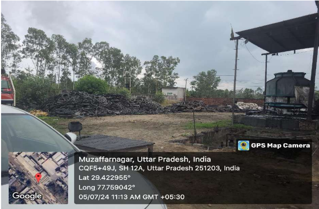
Figure 1 Unit premises entrance without proper gate and hoarding
