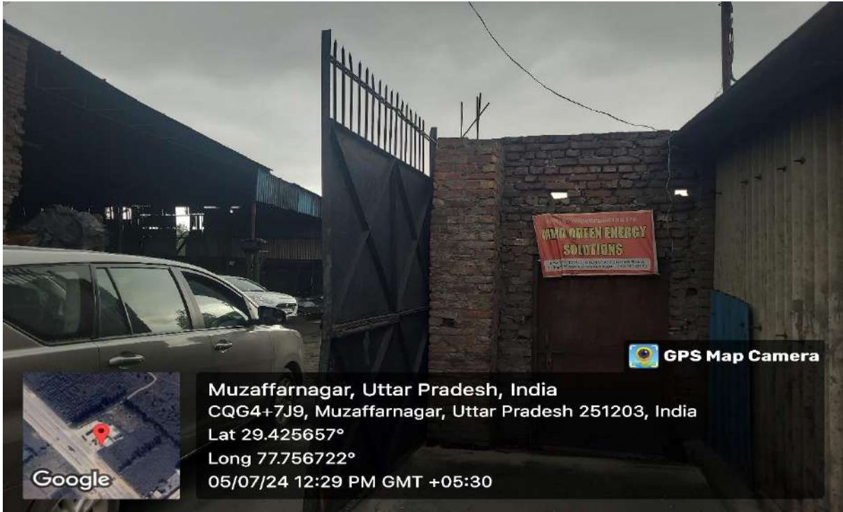
Figure 1 Unit main entrance gate
