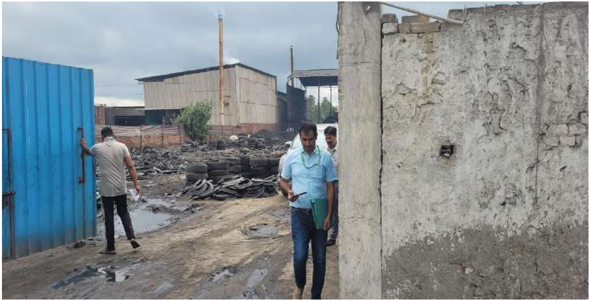
Figure 1 Main entrance gate of the Unit
